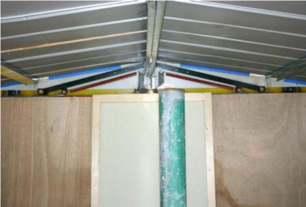
Rear view : First mount the internal springs and the levers.
