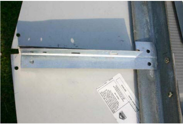
Preparation of gables for setting up of the tilting mechanism.
