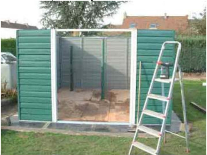
Rear View. The plastic is placed on the ground followed by a sheet of insulating polymer fabric. Then the floor frame is assembled and bolted into the concrete with dowels. The polystyrene plates are cut and placed in the cells and then the wood floor is cut according to the manufacturer's specifications. We must think about making the cuts crossing of pole also accurately as possible (for me, the diameter of poles + 2 inches). We can if we have finished, filling this space with foam rubber (gasket car door). Front view, the four walls, the floor is installed. With using a cordless drill, it is easy to assemble. The rigidity of the construction is remarkable. I also planned to double walls with polystyrene and plywood. This will be next spring when the weather permits. But first, we must think about the final arrangement, and the passage of electric cables for supplying the telescope, lighting, computers and anything that may be necessary to spend the evenings.
