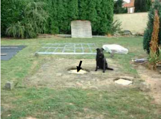
The work just started, already the guardian of the field has laid the first stone to the edifice. In this case, her hedgehog. But it is obviously for play ... One of the two visible holes in the previous picture which will each receive a galvanized steel pole 125mm in diameter. The first will receive my mount tracking for taking photo and the other my EQ5 and perhaps an EQ6... It is not prohibited to dream.
