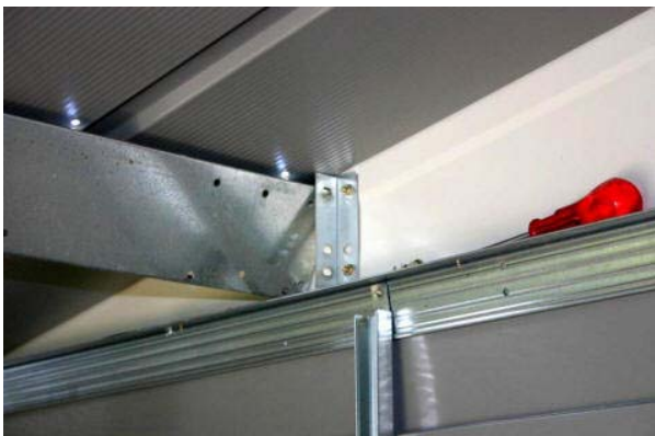
Placing beams on the middle of panels.
