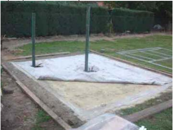
You can see in the foreground, the floor frame and the plastic sheets to isolate the building to the ground. I used rafters to mark the perimeter of the area of the site and raise the shelter. See the rafters on this photo, frame reinforced concrete, soil tamped and the gravel.
