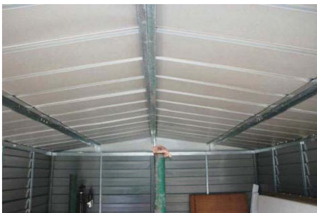
Overview after reversal of the roof beams in the mid-panels.
