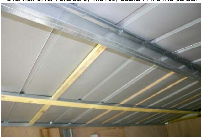
Setting up the wood batten for making slide panel.
