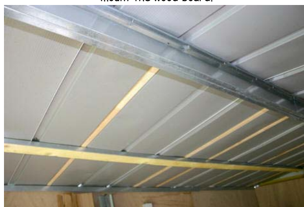
Strengthening beams and panel.
