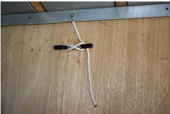
Viewed on fixation of the roof with a mooring cleat.
