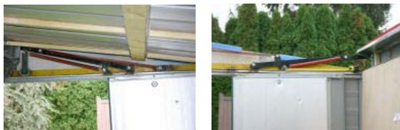
The springs open and closed position.
