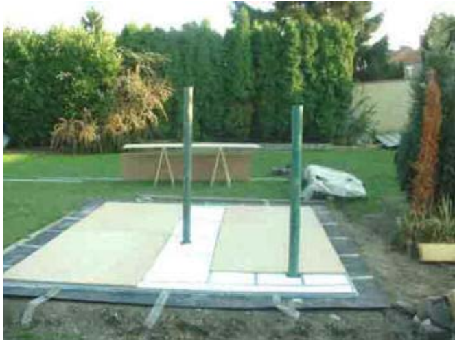
Rear View. The plastic is placed on the ground followed by a sheet of insulating polymer fabric. Then the floor frame is assembled and bolted into the concrete with dowels. The polystyrene plates are cut and placed in the cells and then the wood floor is cut according to the manufacturer's specifications. We must think about making the cuts crossing of pole also accurately as possible (for me, the diameter of poles + 2 inches). We can if we have finished, filling this space with foam rubber (gasket car door). Front view, the four walls, the floor is installed. With using a cordless drill, it is easy to assemble. The rigidity of the construction is remarkable. I also planned to double walls with polystyrene and plywood. This will be next spring when the weather permits. But first, we must think about the final arrangement, and the passage of electric cables for supplying the telescope, lighting, computers and anything that may be necessary to spend the evenings.
