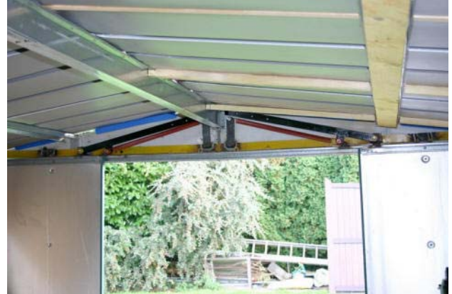
Front panel : the levers and the internal springs mounted.
